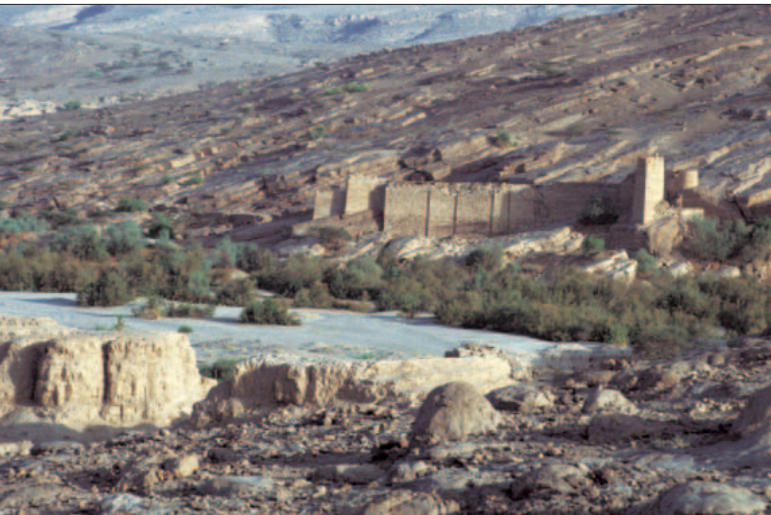
An ancient dam. Without it, the Kingdom of Sheba would not have existed for long.
